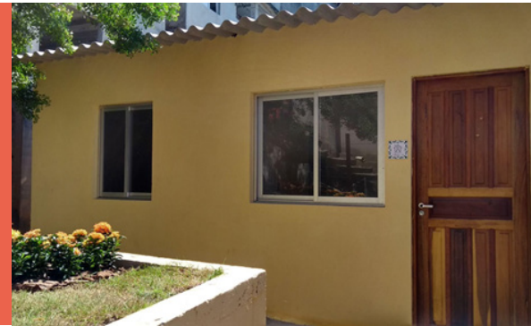
Figure 101: Front facade of Maria Sonia's residence after renovation. Source: Ivan Rocha.
