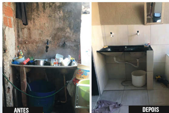
Figure 66: Improvements in housing: a healthier home prevents numerous diseases. Photo: CODHAB DF.
