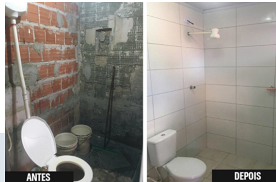
Figure 65: Before and after ATHIS. Source: CAU/RS collection.
