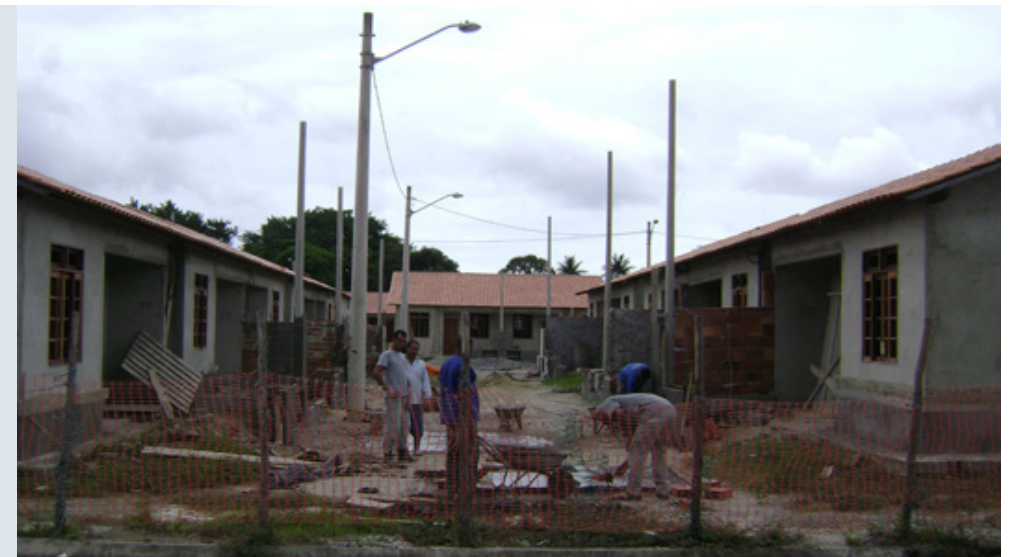
Figure 53: Final phase of the work of Conjunto Esperança in 2015. Source: https://rioonwatch.org.br/?p=44304
