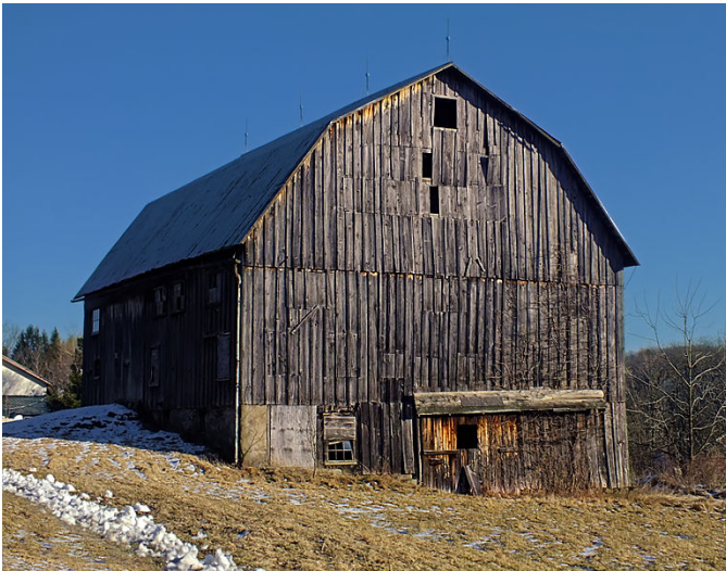
Barn with gambrel-style roof
