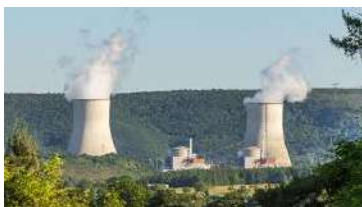
Figure Figure 7.2.2: The Chooz Nuclear Power, in a valley in Ardennes, France, is a reminder that human activity impacts the planet greatly.
