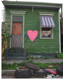
Figure 13.6.4 - House in New Orleans
