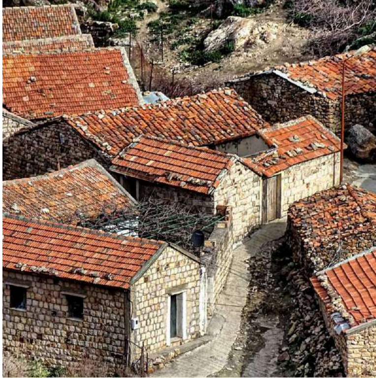
FIGURE 3.3 These houses in Northern Algeria, built by the Kabyle people, are constructed of stone, and include open space for both animals and human inhabitants under a shared roof. (credit: PhR610/flickr, CC BY 2.0)
